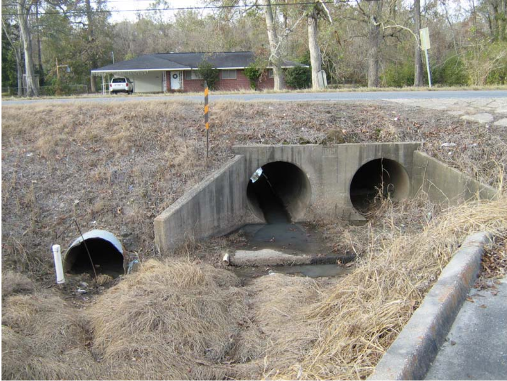
Northerly view of Drainage Feature 2
