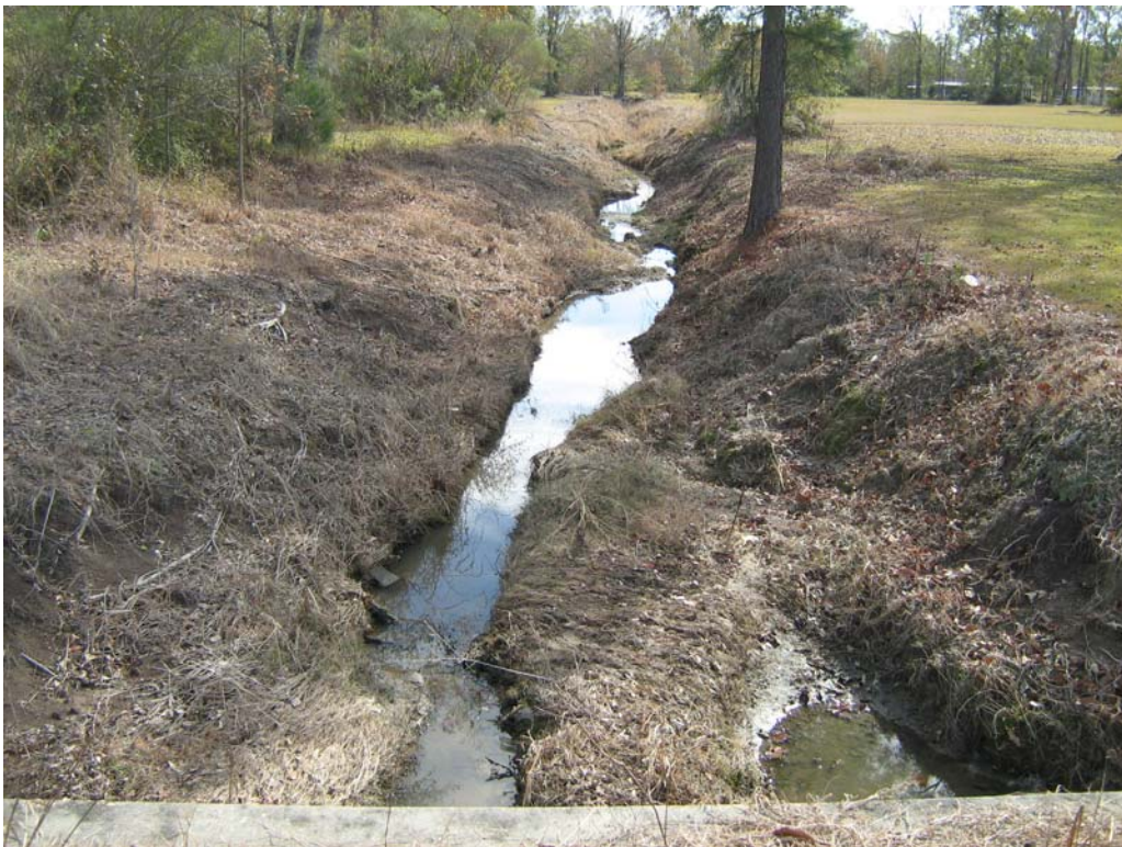
Southerly view of Drainage Feature 1
