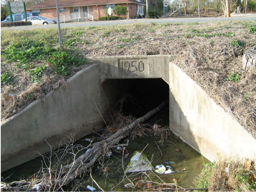
Northerly view of Drainage Feature 3
