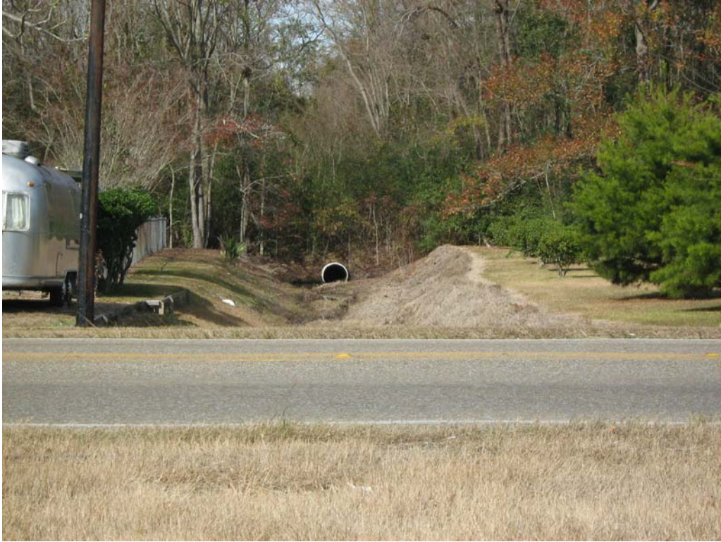
Northerly view of Drainage Feature 1
