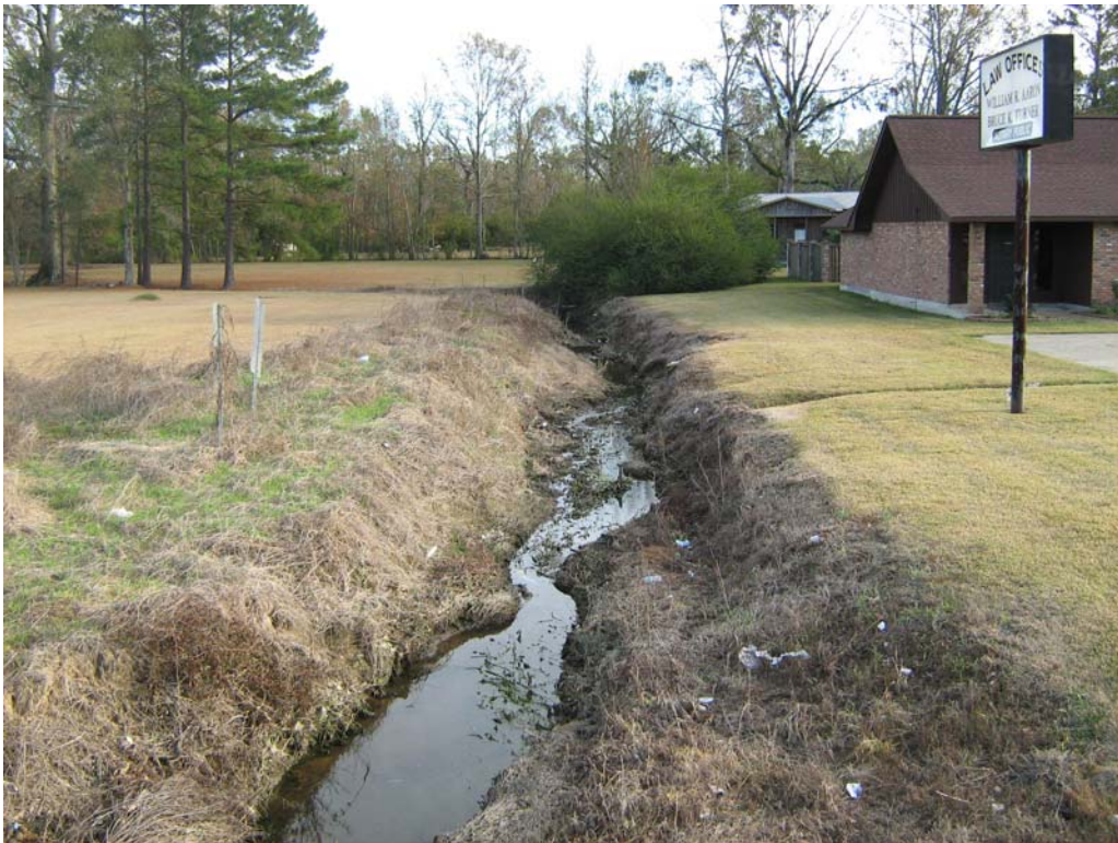
Southerly view of Drainage Feature 4
