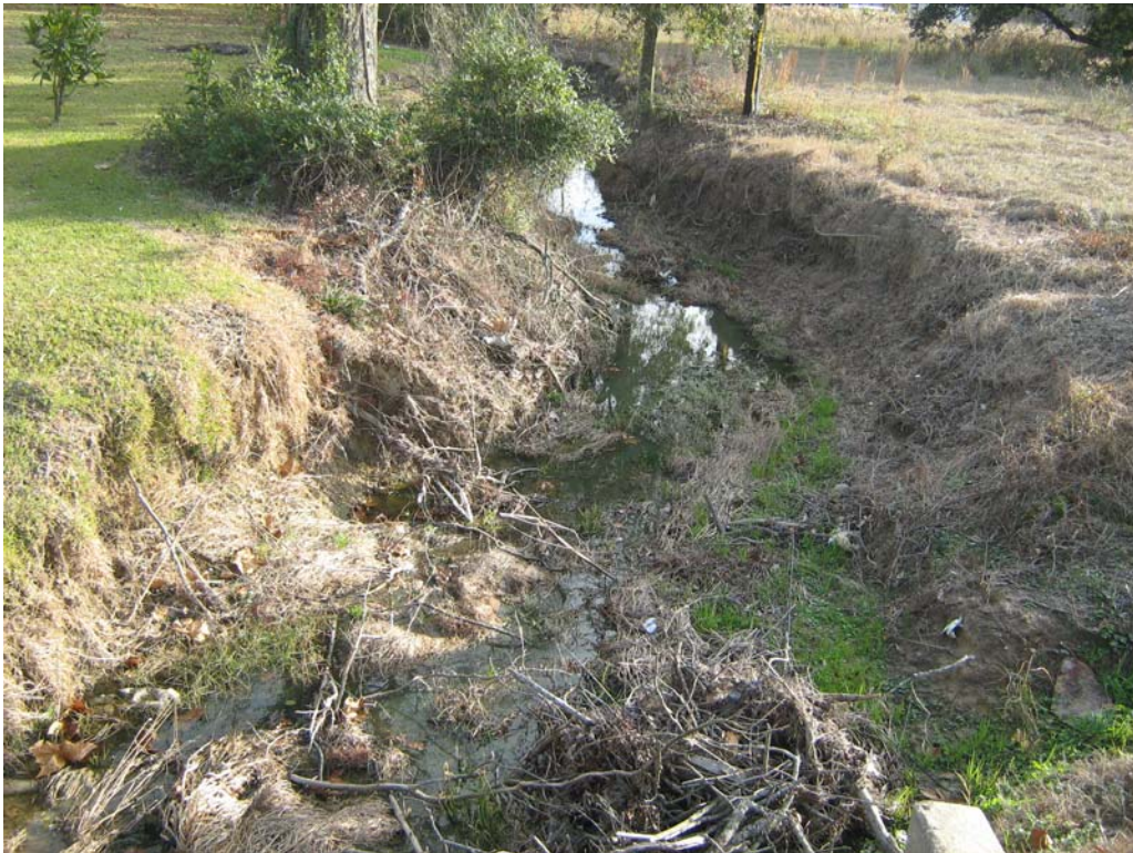
Southerly view of Drainage Feature 3
